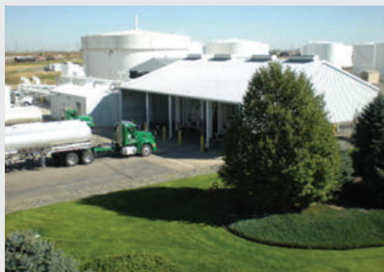
Truck loading facility.
