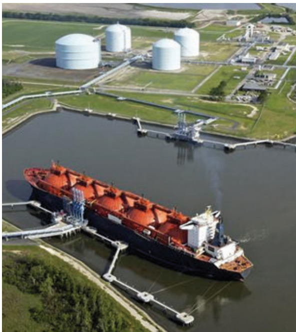
Insulated Low Pressure Storage Tanks for LNG
