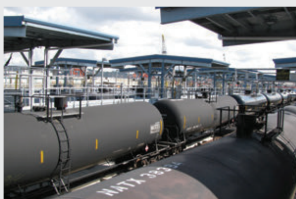
Rail loading facility.
